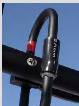
Sealed feed point
